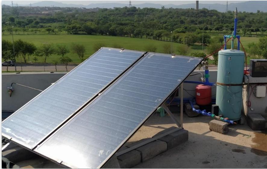
**Fig. 2: EFPC system with calorifier, expansion vessel, data logger and control unit in the background**
