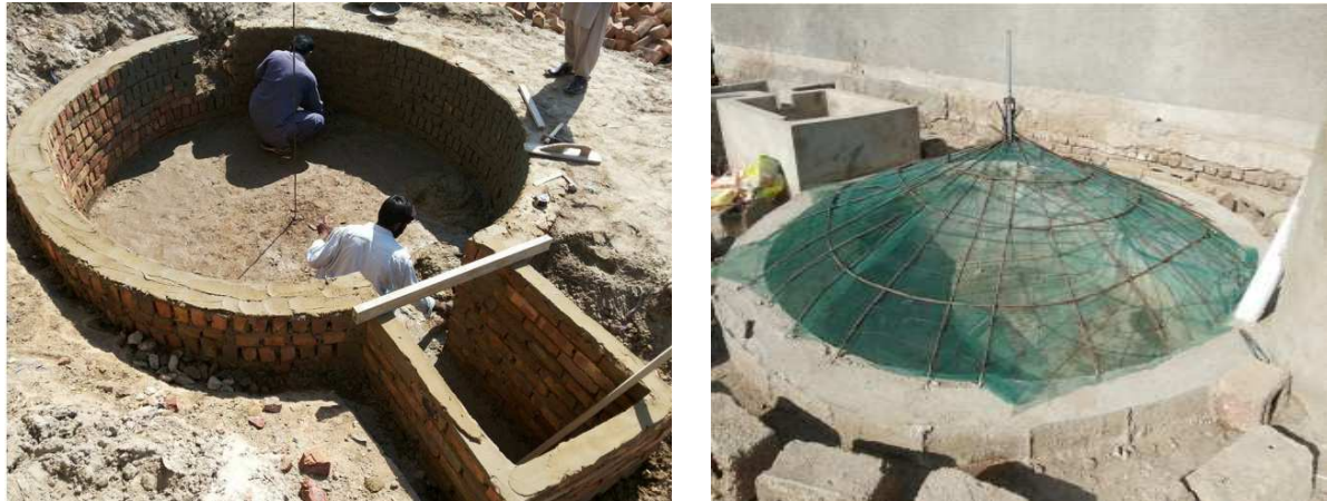
Fig. 3. Construction of Dome
