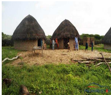
Fig. 4. District Tharparkar after the Rain (houses after rain)
