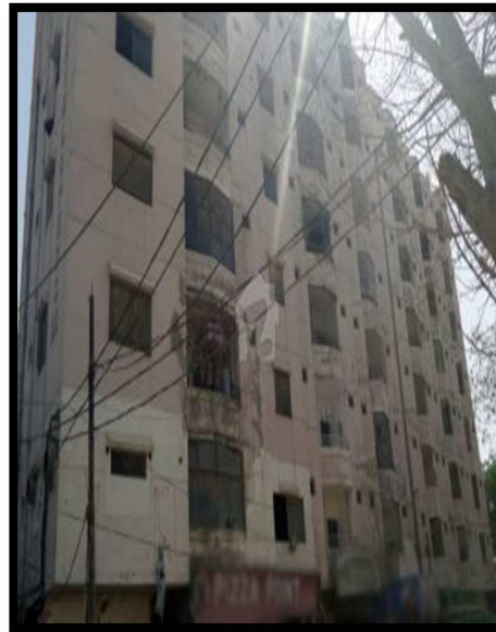
(g) Figure:7 External view of building environment
