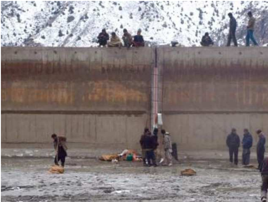
Figure 2.4 Construction site of Naltar Hyde power plant
